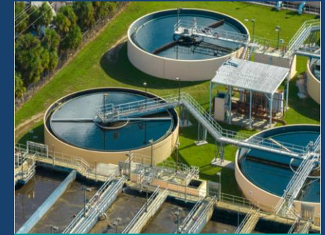
Water & sewage treatment
